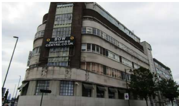
Fig. 1.15: Bow House Business Centre
